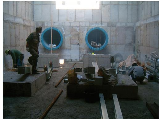
(f) Installation of turbine base concrete
