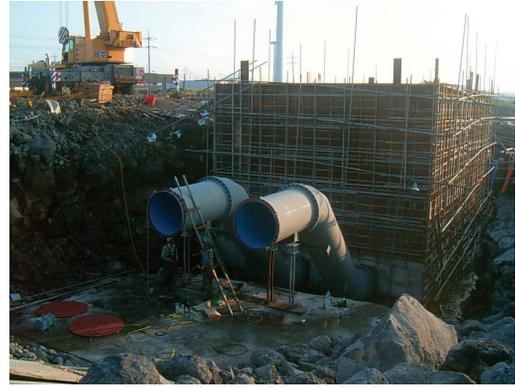
(e) Wall curing and installation of inlet tube
