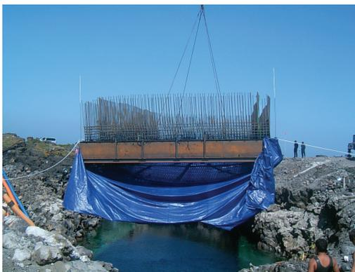
(c) Installation of concrete base
