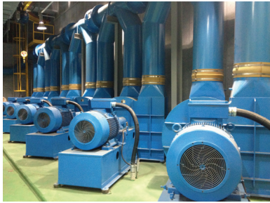
Fig. 2 Blower system installed at the domestic site of a automated vacuum waste collection system
