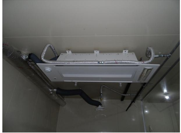
Fig. 15 Chilled beam unit installed in ceiling
