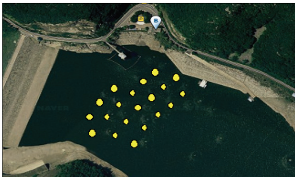
Fig. 8 Installation of water aeration
