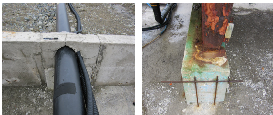
Fig. 2. Status of oil storage tank
