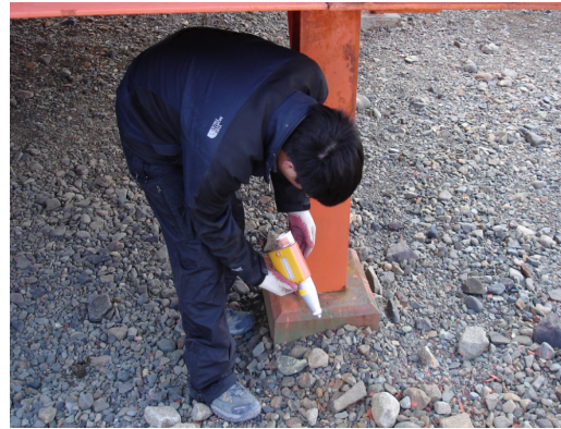
Fig. 3. Schmidt hammer test appearance
