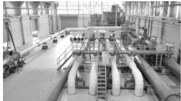
(b) Photograph of facility
