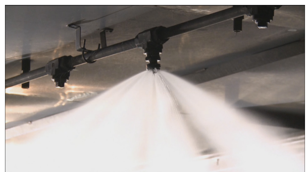
Fig. 4 Water-mist spray of nozzle C
