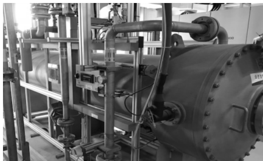
Fig. 4 Photograph of ozone generator
