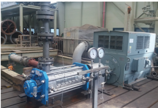
Fig. 8 Pump test facilities
