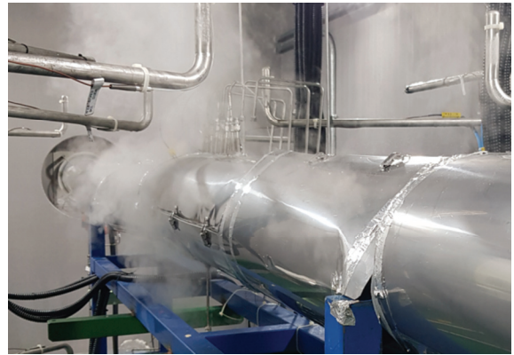
Fig. 13 Leak detection test (70 bar steam, 0.23 gpm)
